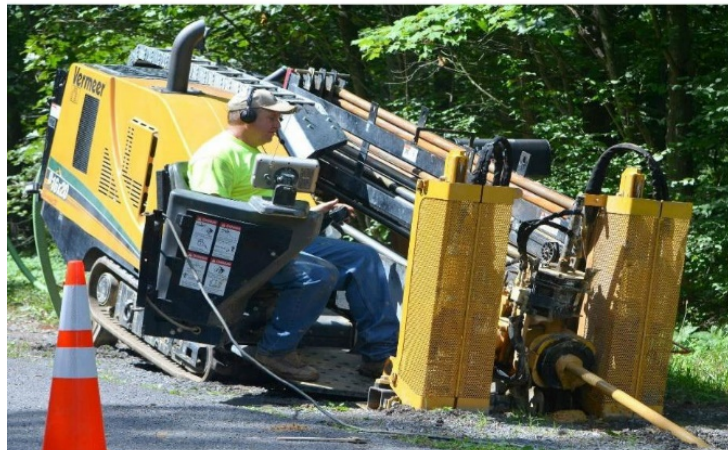
Figure 7: Fiber Installation Continues in Hampshire County
